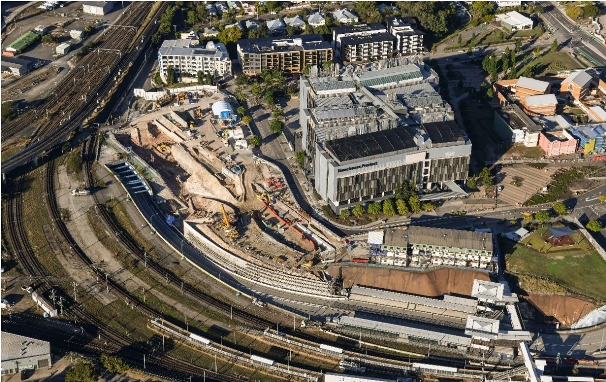
Figure 1 Aerial progress at Boggo Road worksite, August 2020
